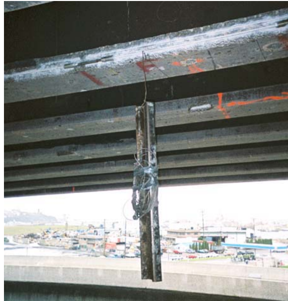
Photo 6. Deflection Test Dead Weight
