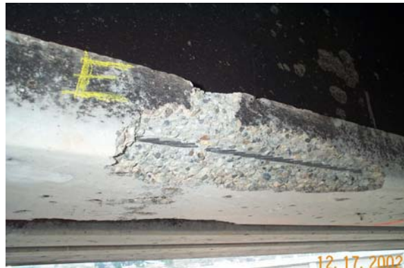
Photo 5. Buff Color Concrete Girder 8E
