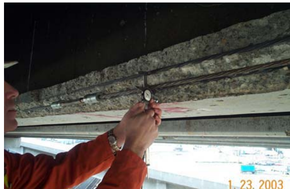
Photo 7. Deflection Test Measurement
